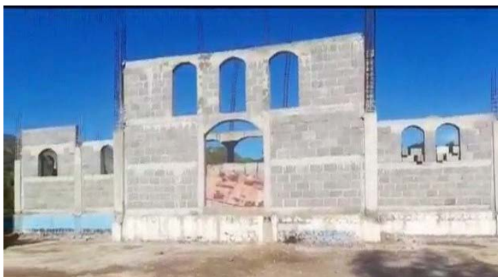
New "Above Ground Church" construction
