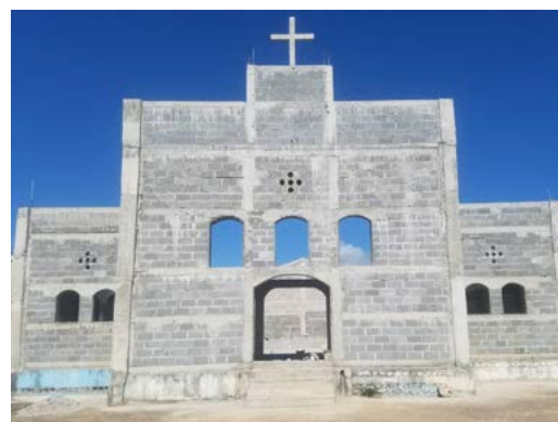
Ste. Marie-Madeleine Church under construction.
