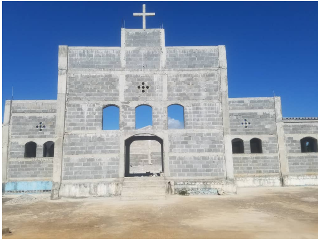
Ste. Marie-Madeleine Church under construction
