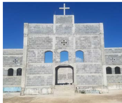
Ste. Marie-Madeleine church under construction.
