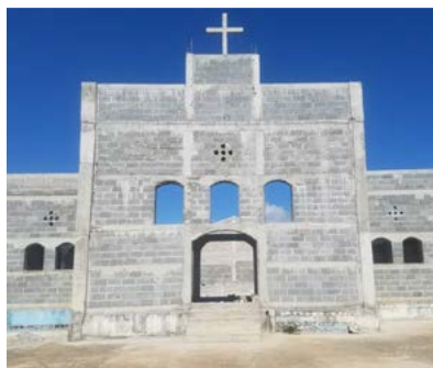
Ste. Marie-Madeleine church under construction.
