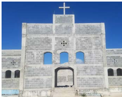
Ste. Marie-Madeleine church under construction.
