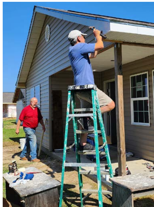
Habitat home under construction.
